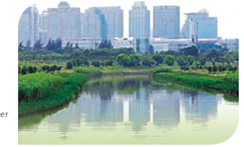
凤塘河主河道修复后 After Fengtang River reconstruction
